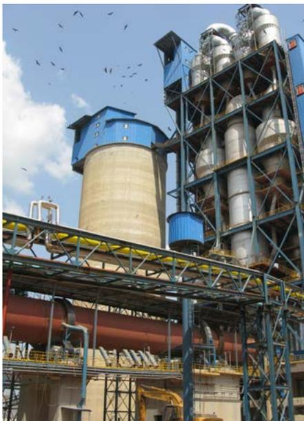
Using these modern heat recycling systems in this way, we can heat the raw material to about 900C before it
